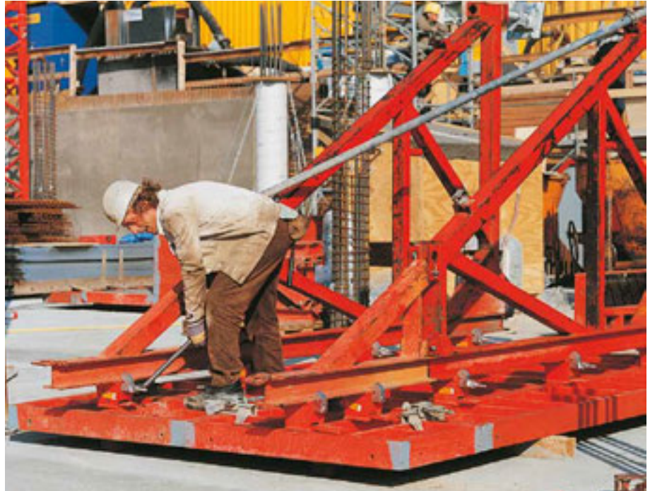
Assembly of Brace Frames SB-A, B and c on horizontal TRIO elements.
