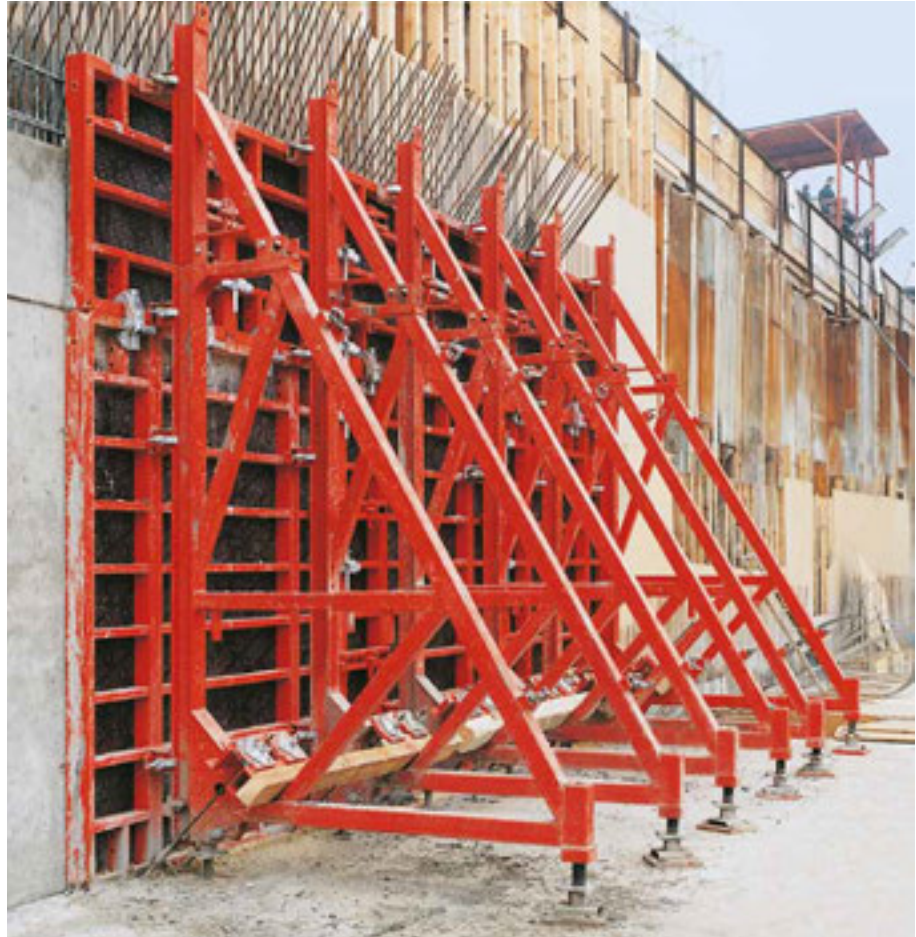
SB-B and SB-C brace frame units with PERI TRIO panel formwork, concreting height 3.50 m.
