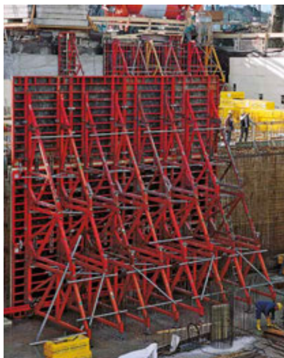
8.75 m concreting height with Brace Frame SB-A0, A, B, C and TRIO.
