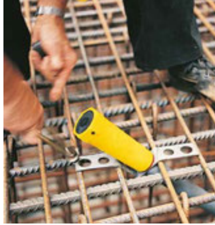
Easy and simple fixing of the anchoring to the reinforcement ...
