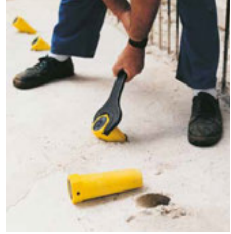
... and easy dismantling of the leading anchor coupler.
