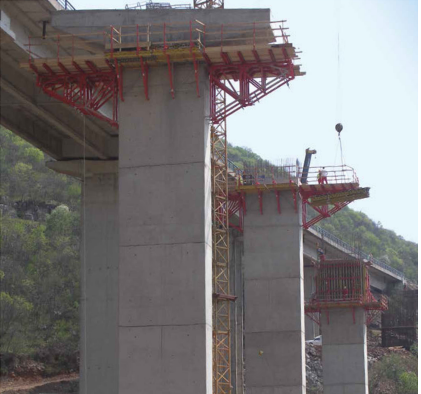
Using SB-A and B brace frame systems as working platform and heavy-duty brackets.
