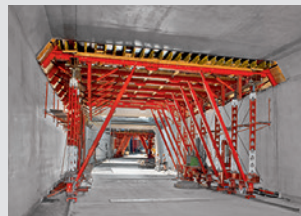
Tunnel Formwork
