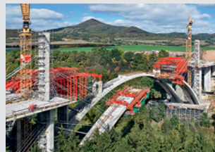
Bridge Formwork
