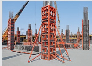
Column Formwork
