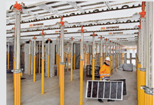
Slab Formwork
